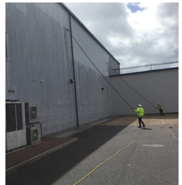
Use of reach & wash system
