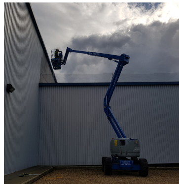
Use of high level access equipment
