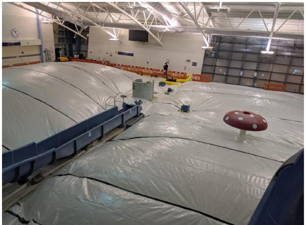
**DBK Drymatic II – A unique and patented heat and air exchange drying solution.**
