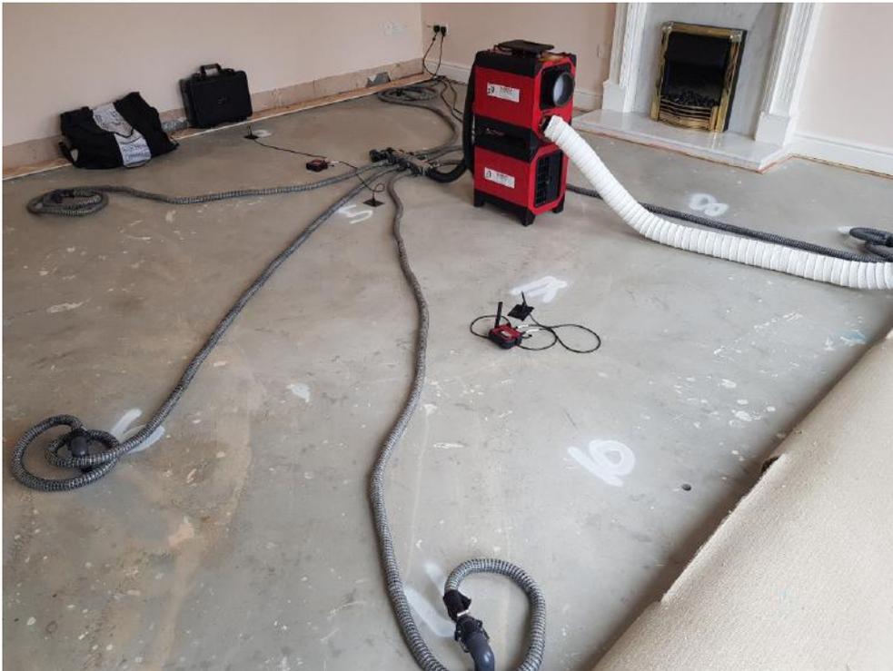
Positive pressure drying is when we take air directly from a desiccant dehumidifier and feed it into a turbine where it is pressurised and driven into the construction through a manifold and a series of 25mm, or 16mm connections.
