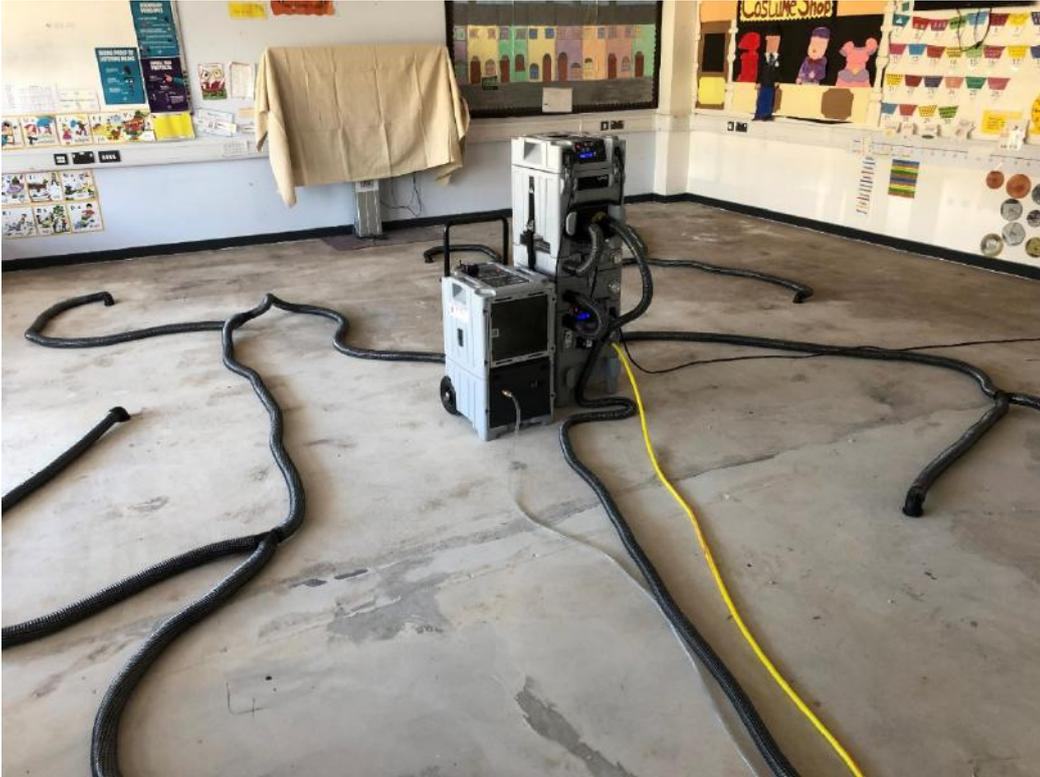
A negative pressure drying solution puts us in full control of the flow of air within a building, ensuring that all air leaving the potentially contaminated sub-floor or cavity space is adequately filtered through a pre-filter and H13 HEPA filter, with the system even having the potential for the installation of an activated carbon filter to manage Volatile Organic compounds (VOCs) and odours on particularly bad claims.
